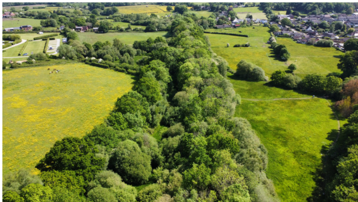
Photo 4 - Aerial view from W looking E along the course of the proposed Trailway on disused railway. Site to right of tree belt.
